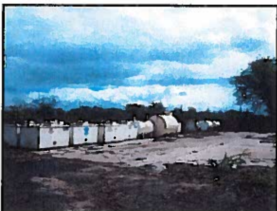
Out of service ASTs located on concrete pad in area of former Building 1569
