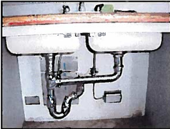
Potential ACM on the underside of sinks at the bathroom facility at Nelson Field
