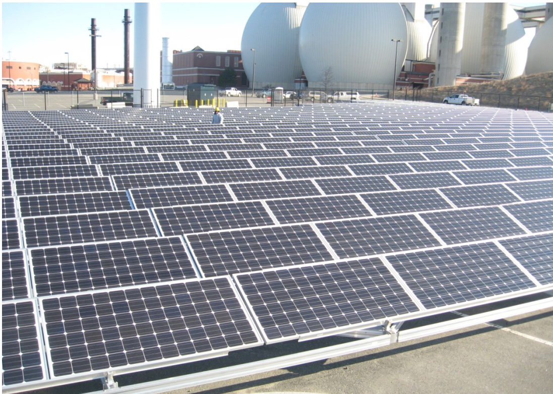
Example of Array Profile and Racking System
